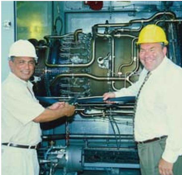
Hon. John Briceno, Deputy Prime Minister, Government of Belize and H. Stanley Marshall, President and CEO, Fortis Inc. at inauguration of the 22-MW Westlake gas turbine in Belize.
