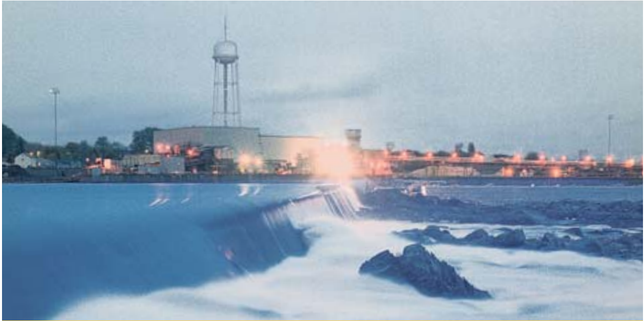
The Exploits Partnership project is a redevelopment of Abitibi-Consolidated's hydroelectric facilities in central Newfoundland.
