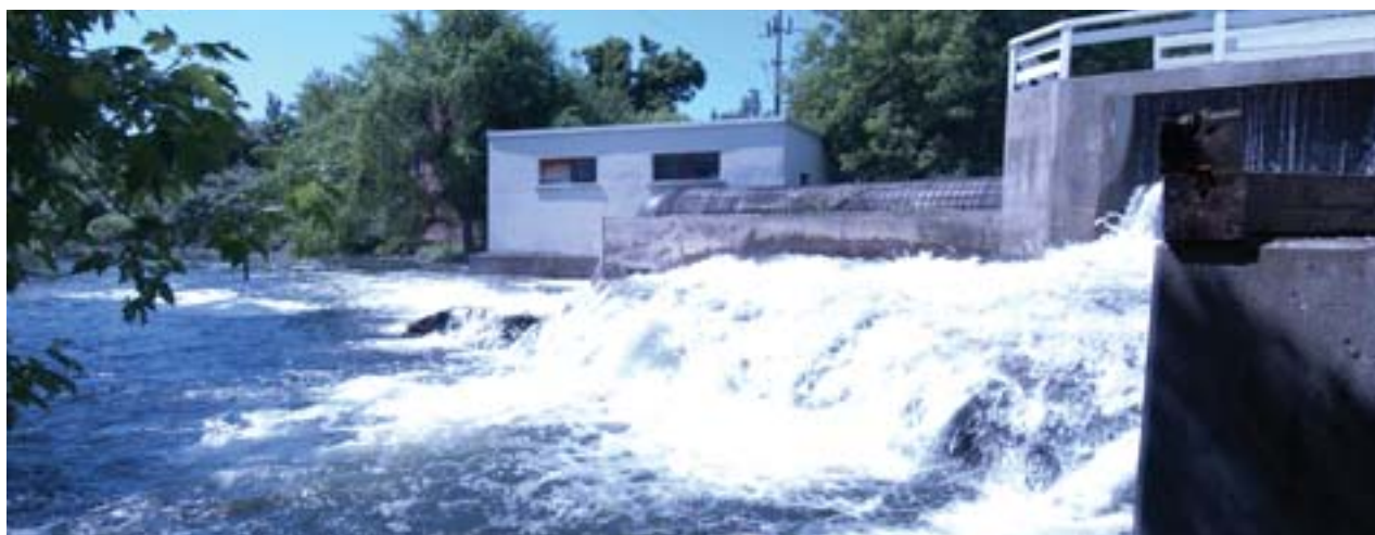
Washburn hydroelectric generating station, Rideau Canal.
