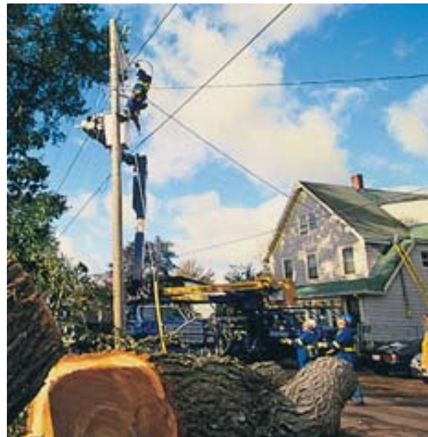
Employees work to restore power to customers impacted by Hurricane Juan.
