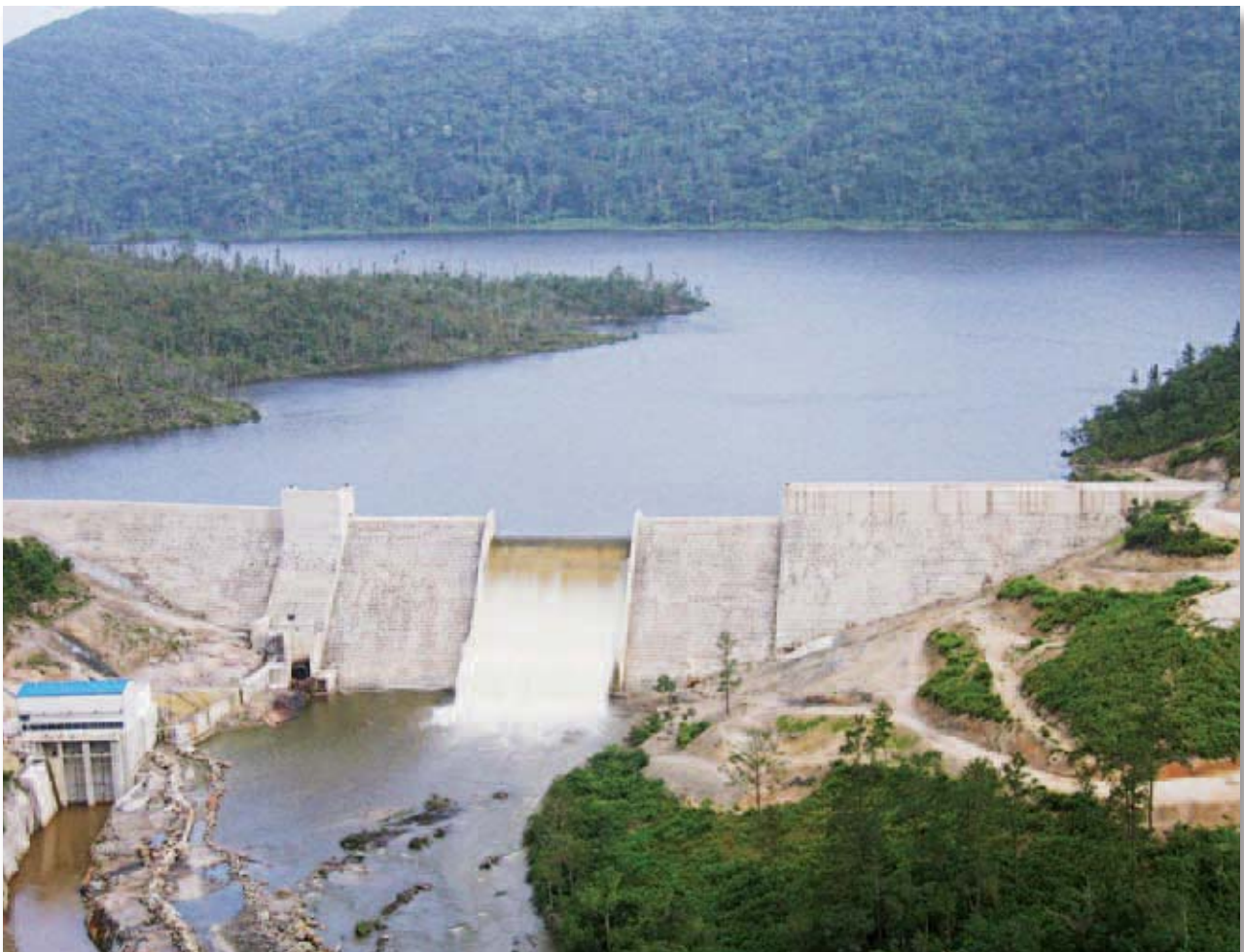
The Chalillo hydroelectric facility in Belize considerably minimized the impact of flood waters in San Ignacio after heavy rains.
