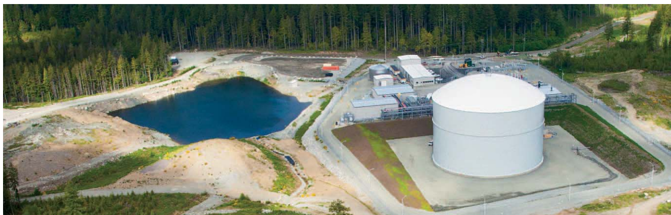
Construction of the $212 million 1.5 billion-cubic foot liquefied natural gas storage facility on Vancouver Island was completed in 2011.
