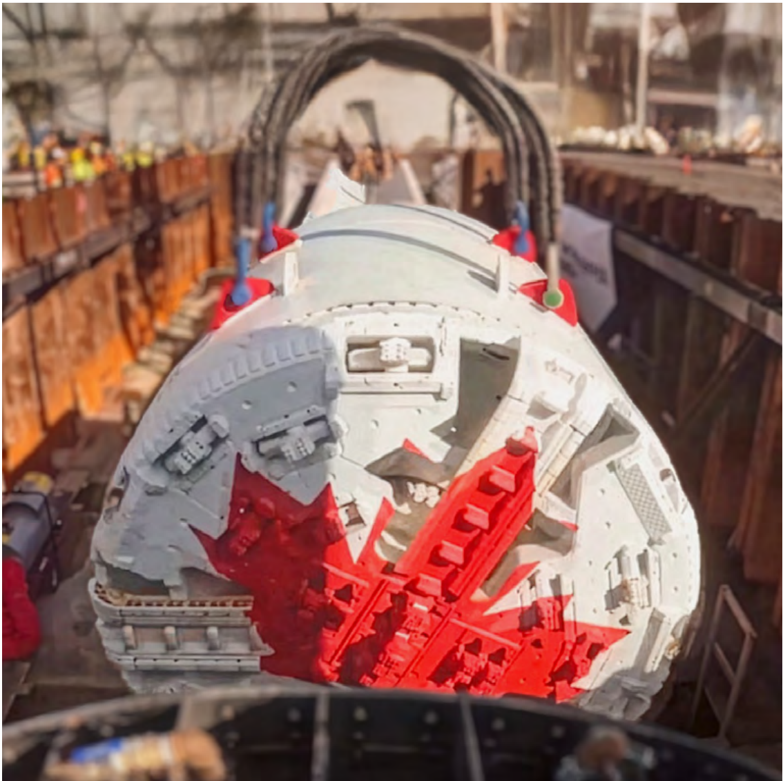
Tunnel boring machine being used to construct a tunnel below Skwelwil'em Squamish Estuary Wildlife Management Area.
